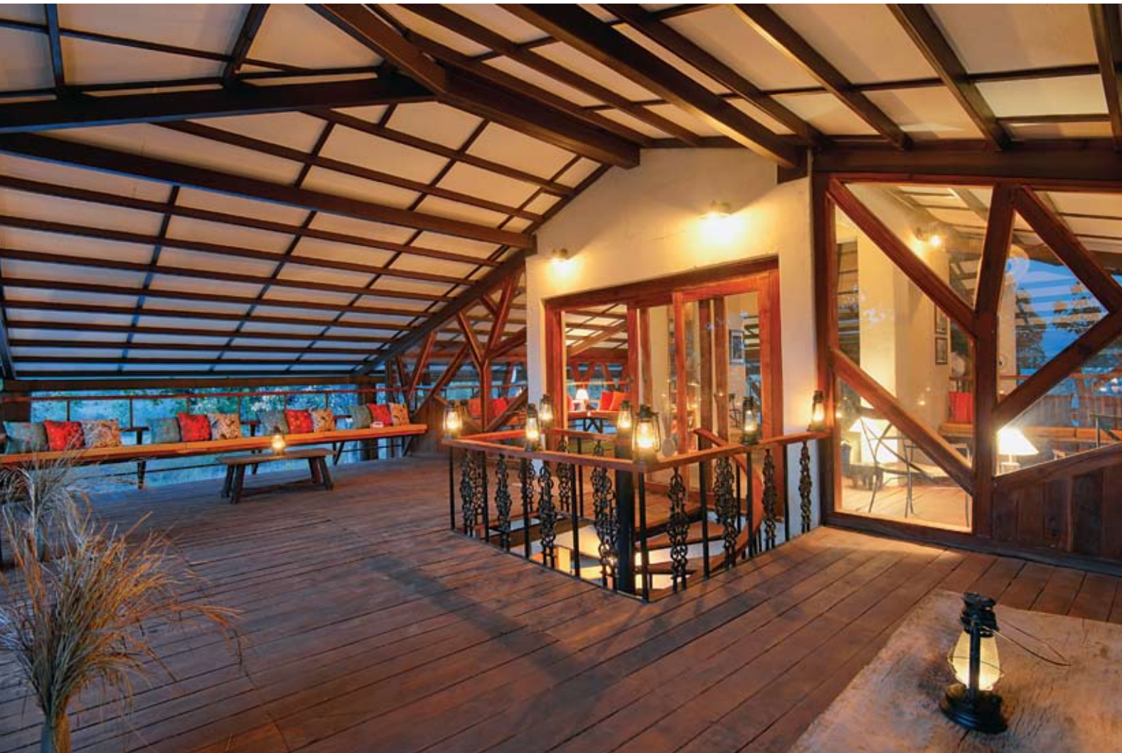
Upper deck lounge of the main building. The floors and roof rest on raw Mahua tree trunks.
